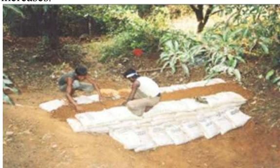
Vanrai bandhara are constructed just after the last rains to arrest the runoff and store water .For few months into the dry season. The typical height of a vanrai bandhara is about 0.8 m to 1.2 m. Length of the bandhara ranges from 6-7 m up to 25 m. The breadth of the bandhara is about 2 m to 2.5 m. The bags used for the vanrai bandhara are 40cm x 30cm x 15cm (l x b x h).
