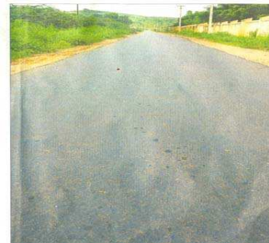
Polymer-Aggregate-Bitumen Mix Road at Madurai, Tamil Nadu Undamaged By Heavy Rain
